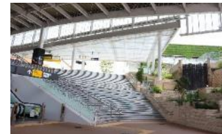
A rainwater storage facility under the large stairs and a planting with highly efficient watering equipment
