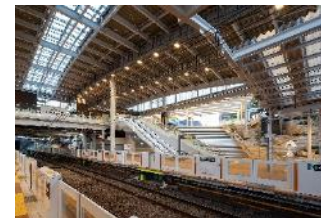
Minami-machida Grandberry Park Station
