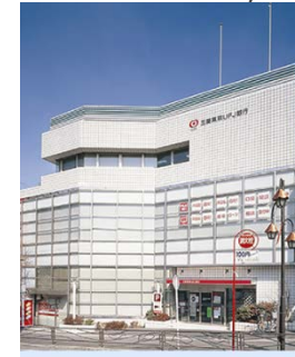
Tokyu Saginuma No. 2 Building
