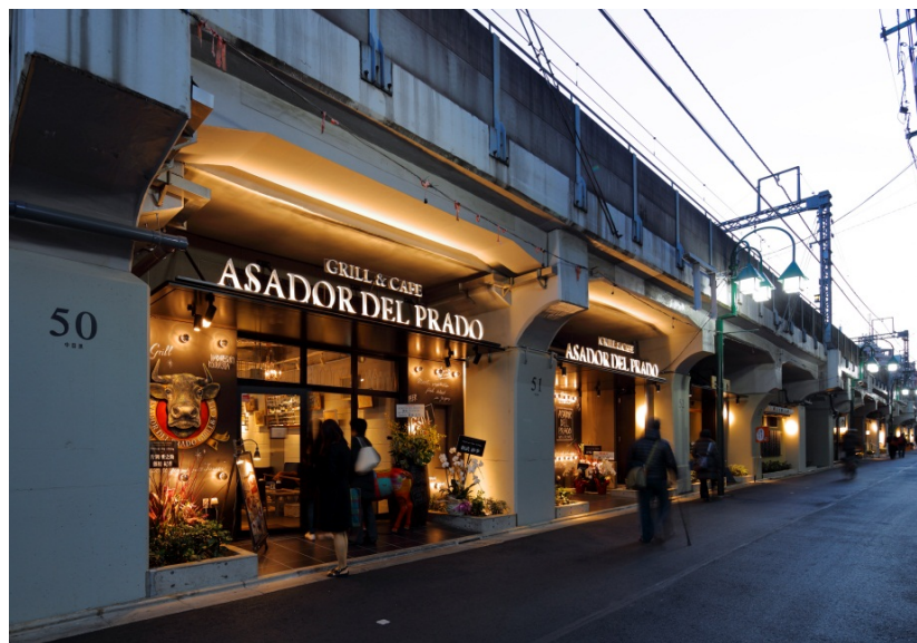
▲ Underneath Naka-meguro Station Site area: Approx. 8,300m 2 Approx. 28 stalls opened in an area approx. 700m in length beneath Naka-meguro Station
