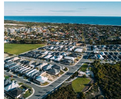
Housing land development project in the Two Rocks area of Yanchep, Western Australia.
