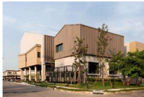
HarmoniQ Residence Sriracha
