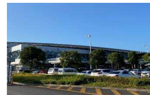
Hiroshima International Airport passenger terminal building
