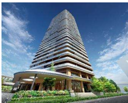
DRESSER Tower Minami-Machida Grandberry Park
