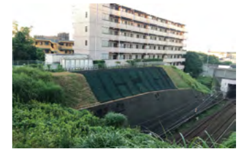
Slopes after countermeasures, between Saginuma and Tama-plaza Stations
