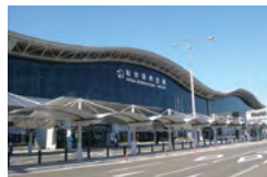
Sendai Airport Passenger Terminal
