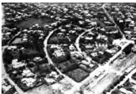
1932 Tamagawa-dai (Den-en-chofu) residential district
