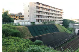
Slopes after countermeasures, between Saginuma and Tama-plaza Stations
