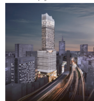
Shinjuku Kabukicho 1-chome Redevelopment Project (scheduled to be complete in FY2022) Site: approx. 4,800 m 2 Total floor area: approx. 87,000 m 2 Use: Hotel, theater, cinema, commercial facilities, etc.
