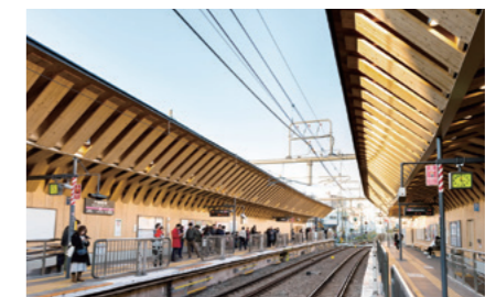
Platforms of the Togoshi-ginza Station
