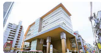
4 Area with anticipated opportunities for business participation, such as the New Airport Line project, and extension of the Gaikan Expressway
