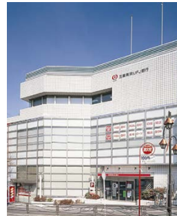
Tokyu Saginuma No. 2 Building
