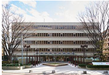
Shin Mizonokuchi Building
