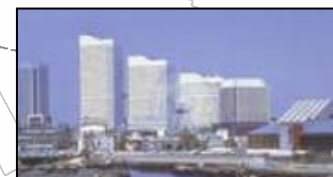
Queen's Square Yokohama (Opened in July 1997)
