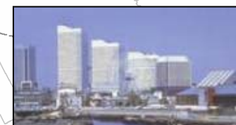
Queen's Square Yokohama (Opened in July 1997)
