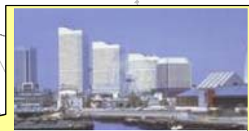
Queen's Square Yokohama (Opened in July 1997)
