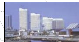
Queen's Square Yokohama (Opened in July 1997)
