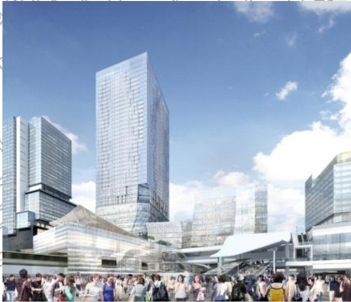
Shibuya Station Block, East building to be opened in 2020
