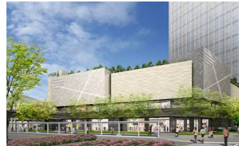
▲ View from Traffic Place Side
