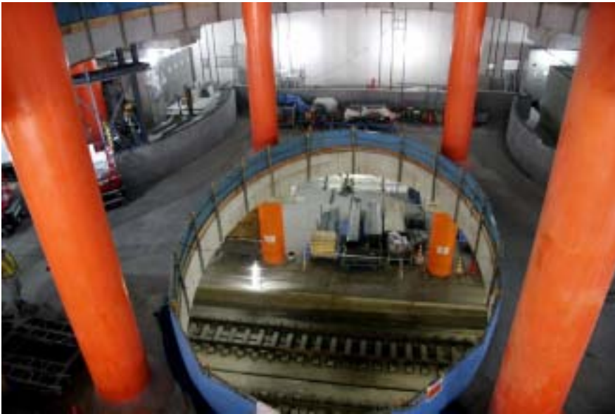
Construction of new Shibuya station
