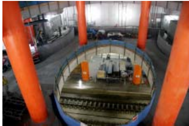
New Shibuya Station (under construction)
