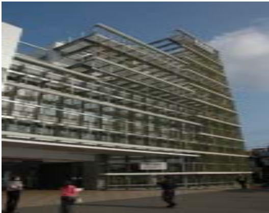
Tokyu Hospital (Ookayama Station)
