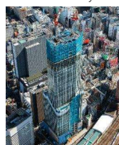
State of construction progress
