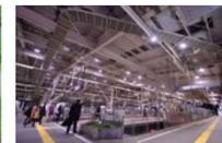
Kamata Station platform lighting replaced with LEDs
