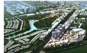
Panoramic View of the Binh Duong New City project
