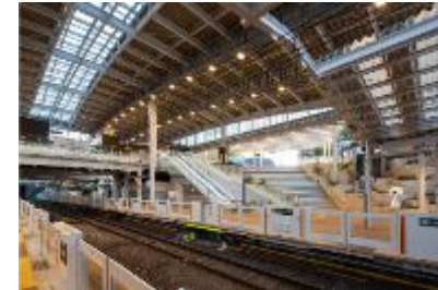
[Minami-machida Grandberry Park Station] Recognized for utilization of rainwater as flushing water for passenger toilets, rainwater drainage plan through the installation of large volume rainwater storage tanks, introduction of LED lighting, and achieving an approx. 70% recycling rate for waste materials generated during construction.
