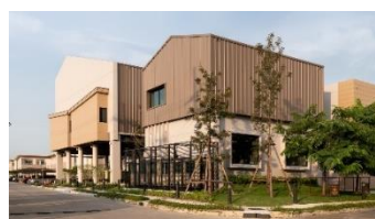
HarmoniQ Residence Sriracha
