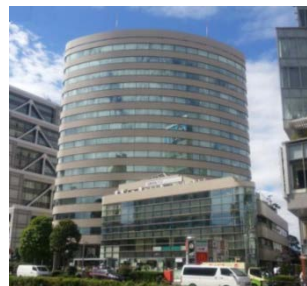
Aoyama Oval Building
