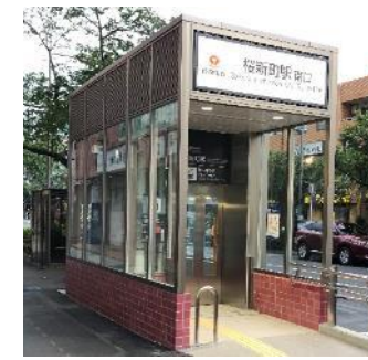
Sakura-Shimmachi Station South Exit elevator (second route)
