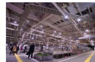
Kamata Station platform lighting replaced with LEDs
