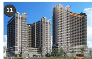
The NEST (施工中)
