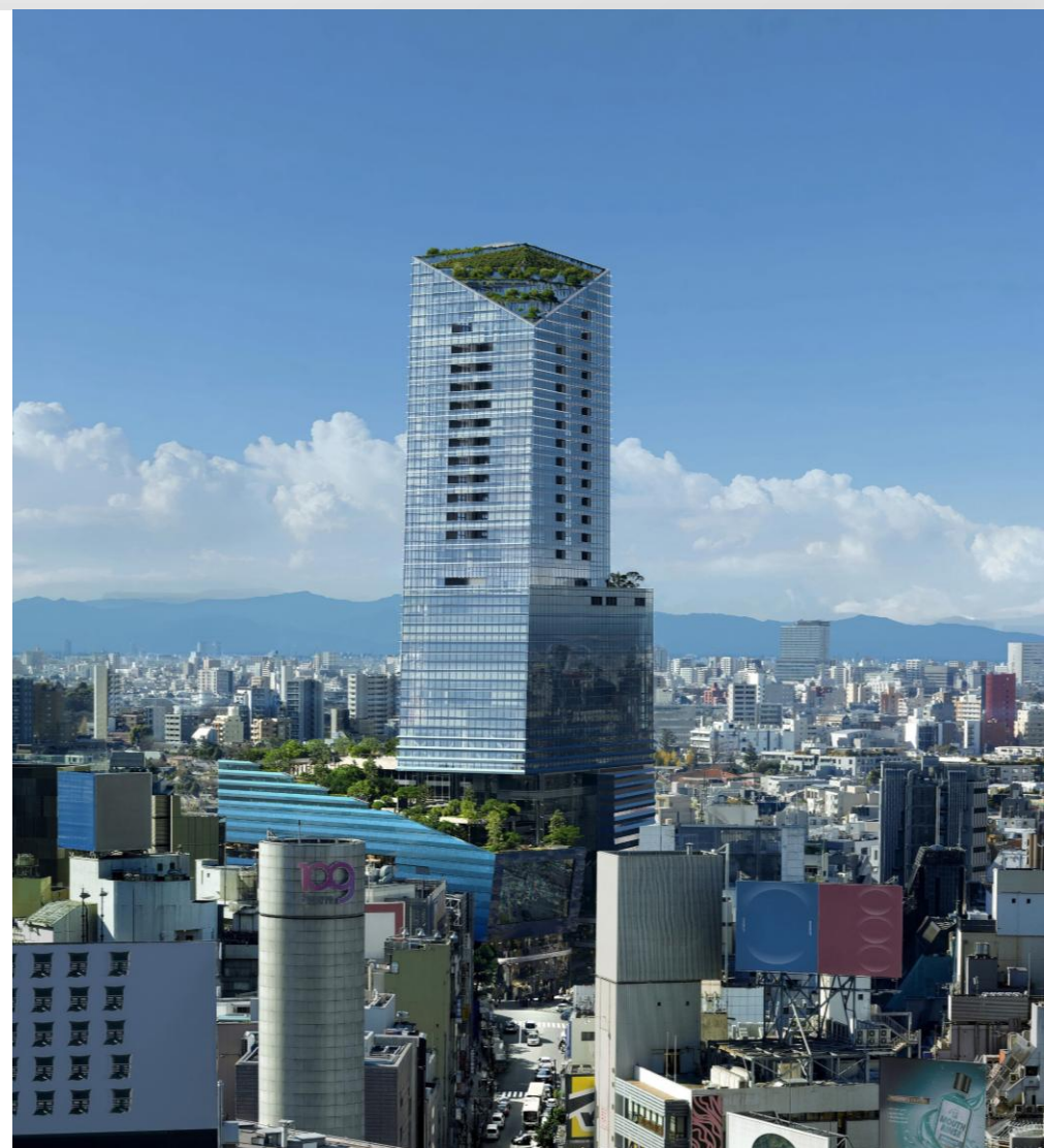
Shibuya Upper West Project 外観イメージ Image by Mir / Copyright : Snøhetta and NIKKEN SEKKEI LTD
